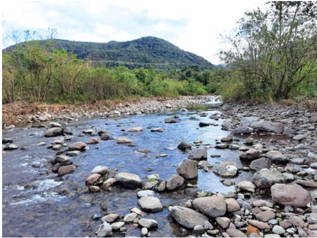
Fig. 8: Photo showing gravel drainage channel. (Source: Beth Rocha)
